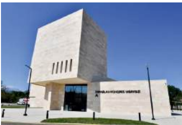
ZANGILAN CONVENTION CENTER COMPLEX
